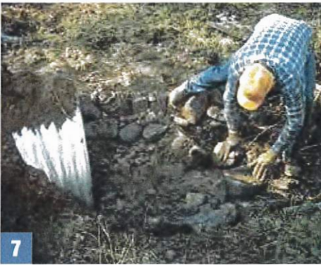
Armor the culvert inlet and outlet. Rocks, logs or grass seeding can be used to protect these locations against erosion. Check the area upstream and downstream from the culvert. Clear upstream area of woody debris that might plug the culvert.
