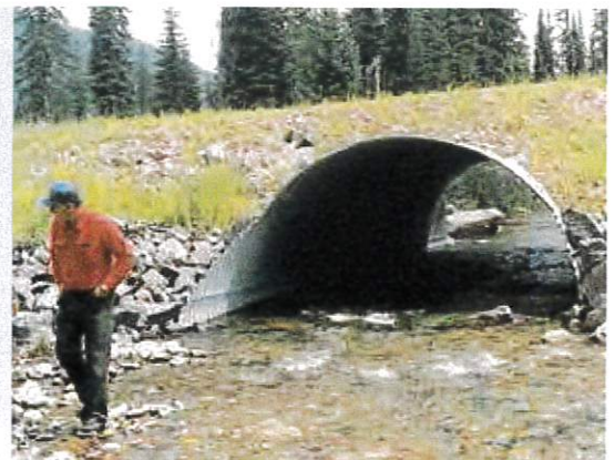
Bottomless arches leave the streambed intact, making it easier for fish to pass. Natural streambed roughness creates pockets of low water velocity where fish can move comfortably. Bedrock or concrete footings are required.
