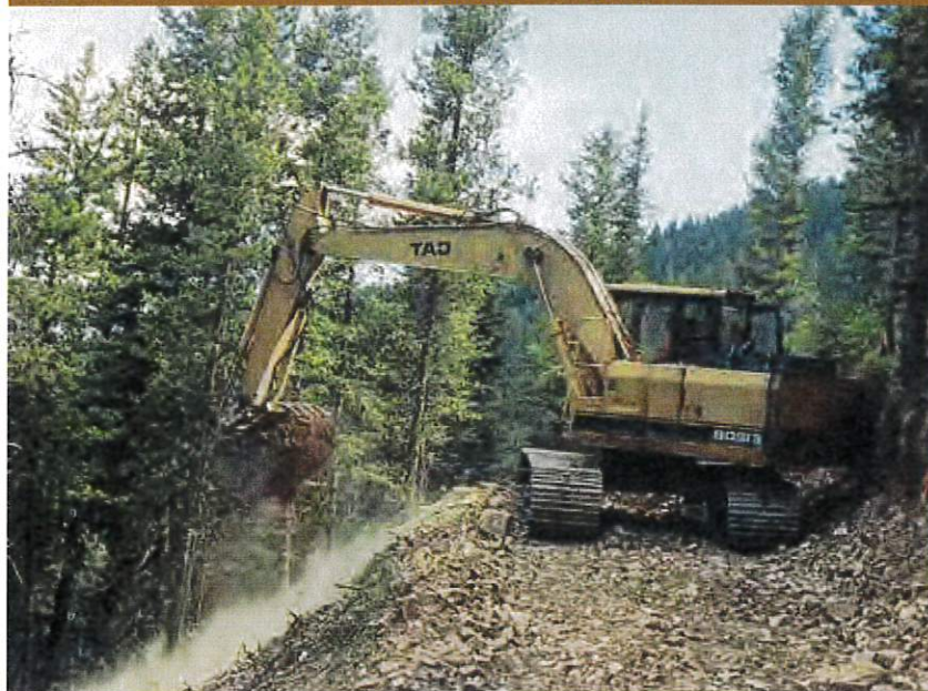
Excavator dismantling the road corridor.
