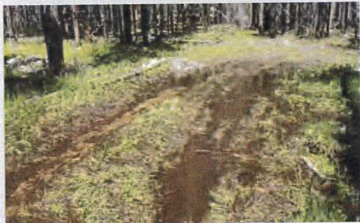
Damage to roads and streams can result from poor crossings and lead not only to washed out roads but to heavy stream sediment loads and damage to streams and fisheries.
