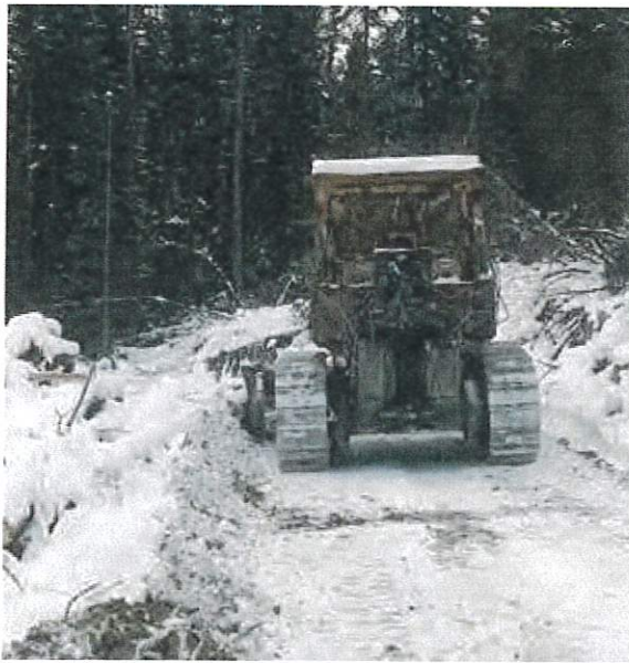
To provide a winter road grade capable of heavy hauling, always remove snow cover. Deep-frozen road surfaces have tremendous strength. Do not let snow cover insulate and weaken the road—plow during cold weather.
