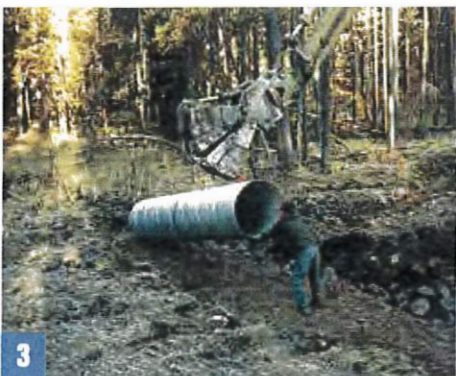
The culvert bed must conform with the natural streambed. The bed should be either rock-free soil or gravel. Bedding should provide even distribution of the load over the length of the pipe. Countersink the culvert to allow stream gravel to deposit in culvert bottom (see detailed diagram, page 40).
