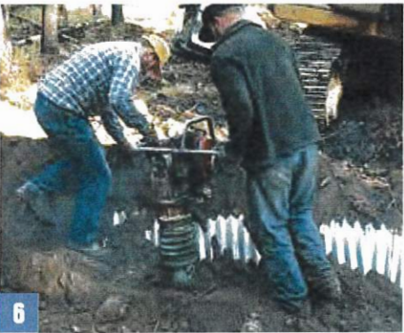
Tamping fill material throughout the entire backfill process is important. The base and sidewall material should be compacted first. This reduces any chance of water seepage into the fill.
