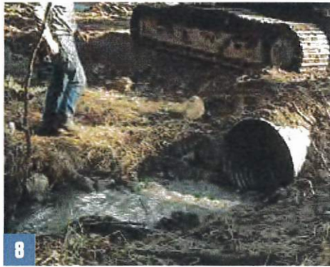
After the new culvert is opened to water, watch for the need for more rock armor. Be sure that a minimum of one foot of compacted soil covers the top of the culvert. For larger culverts, the compacted fill material should be 1/3 the culvert diameter, at a minimum.
