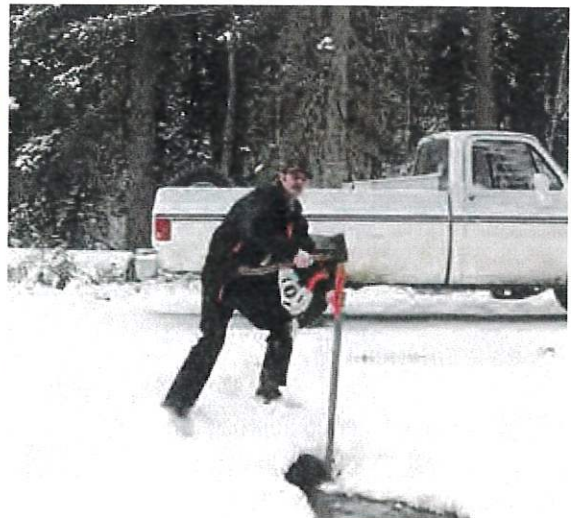
Trying to rely on memory can be expensive when it comes to culvert maintenance. Mark them before the snow falls to avoid logging machinery damage.
