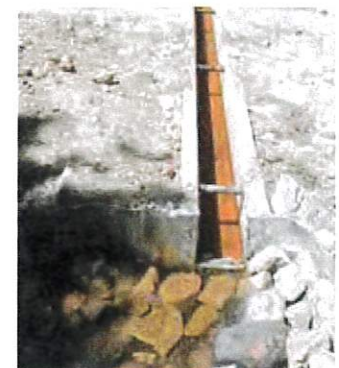
Open Top Wood Culvert
