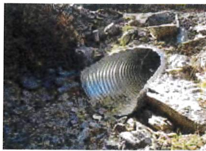
Mitered Relief Culvert Inlets can prevent plugging from soil or debris.
