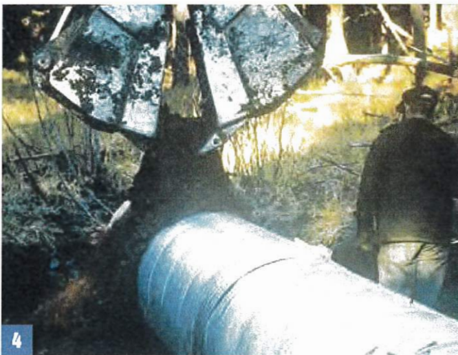
Secure each end of the culvert with backfill. Pour backfill material over the top of the pipe. This allows finer soil particles to flow around and under the culvert sides. Larger particles roll to the outside. Fine soil particles, close to the culvert, compact more easily.
