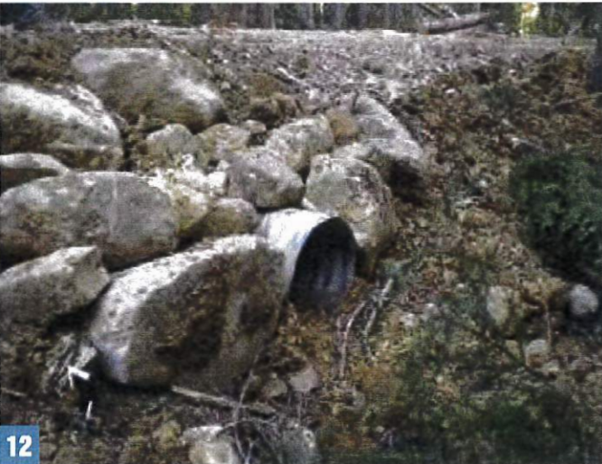
Additional measures that severely limit sediment entering the stream are rock armoring and the placement of a slash-filter window (see page 23) to both limit sediment flow and provide stability to the fill slope.
