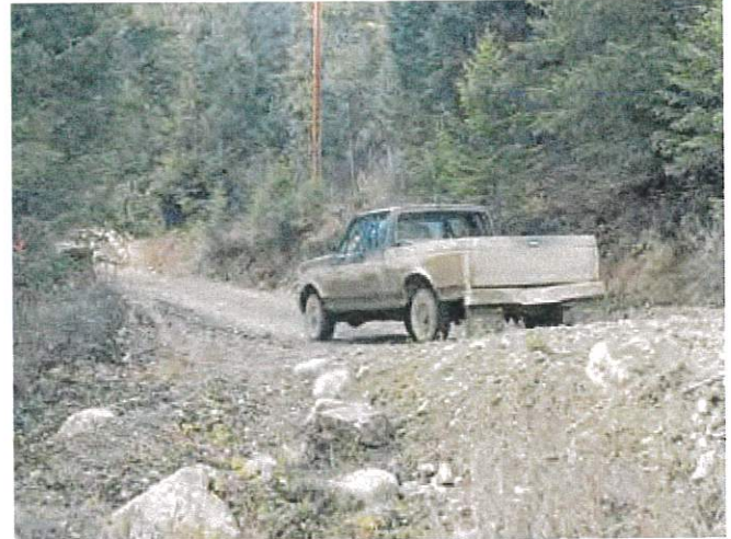
The drain dip bottom is sloped to carry water from the inside to the outside of a road surface and onto natural ground.
