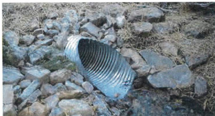
An armored culvert.
