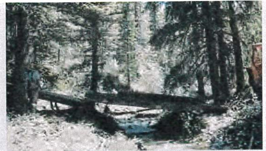
A portable bridge provides access across streams less than 10 feet wide with minimal disturbance to streambanks or bed (310 permit required). Select locations with firm soil banks, level grade, and minimal vegetation clearing.
