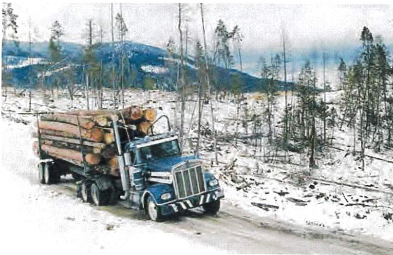
⊘ Road surfaces deteriorate rapidly under heavy hauling and thawing temperatures. This road surface is starting to break up. Hauling should be suspended or limited to colder portions of the day. Standard practice is to begin hauling early, around 3–4am, and stop when the sun softens the road.
