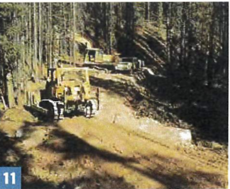
Layers of fill are pushed into place and carefully compacted to build up and maintain a consistent road grade.
