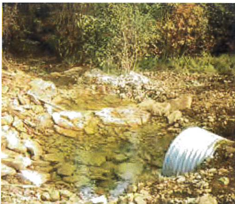
Step pools at culvert outlets can sometimes correct the problem of hanging culverts by allowing fish to rest before attempting passage.
